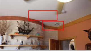
(2) There is moisture impact to the ceiling in the form of stains and or distorted wood COMPONENTS consistent with movement of water movement through the roof deck from precipitation (noted at the sunroom bathroom). These areas should be documented as stabilized by known repairs from a QUALIFIED technician or the roof SYSTEM should be serviced by a QUALIFIED roofing contractor.
