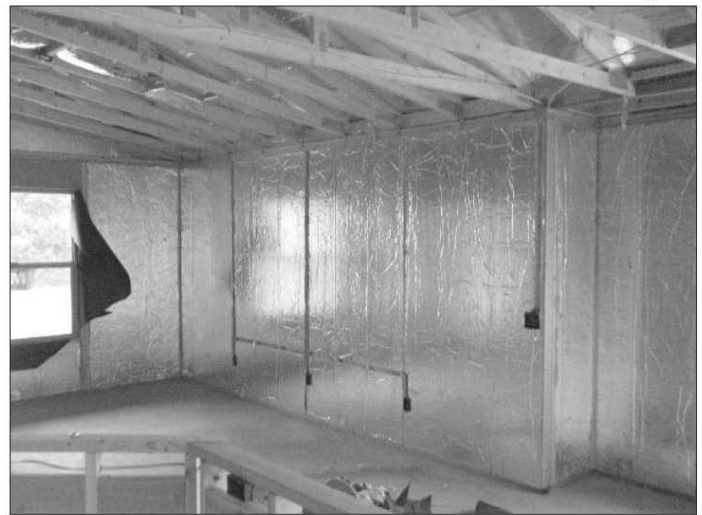
This Silver City Energy Star home is being built by Timberland Construction and uses an inexpensive prefabricated wall system engineered with wood framing at 4-foot centers. The wall sections include rigid high-density insulation to provide R-21 insulating value within an airtight 2-by-4 frame wall cavity.
