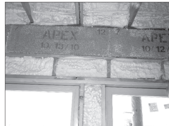
Insulated concrete form walls combined with spray foam insulation fill the attic and wall sections in this David Coyle Home currently under construction and targeting Build Green New Mexico gold certifications in Las Cruces.
