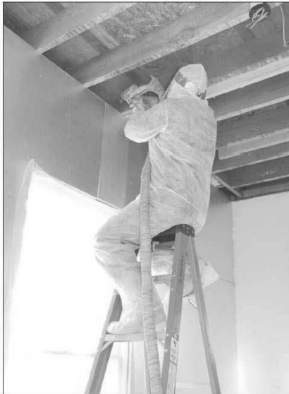
A McGinley Construction worker blows expanding foam insulation into the wall of this proposed Green Build New Mexico home built in 1908 near Pioneer Park. The foam will help provide better insulation.
