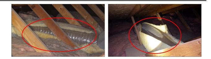
(2) Ventilation ducting is loose and or disconnected within the attic space (noted at each bath fan exhaust duct that terminates in the attic) and should be serviced to extend to a weather protect outlet at the roof or exterior soffit. ACTION RECOMMENDED by a QUALIFIED hvac technician.
